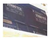
The Bureau believes that the secondary weather barriers whether they are building paper or polymeric-based barriers should be just that...secondary. The primary barrier consisting of metal flashing, caulking and a good Portland Cement Plaster panel, should have characteristics that minimize the amount of moisture that the secondary barrier is forced to handle.
