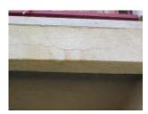
The other type of cracking is the stress cracking that occurs when smooth trowelled stucco is installed. As the sand is compressed into a tight smooth finish, surface stress creates fine, tight, miniature cracks throughout the surface of the finish. This is one of the reasons that the Bureau, while promoting the use of smooth finishes, expects the plaster to be painted.
